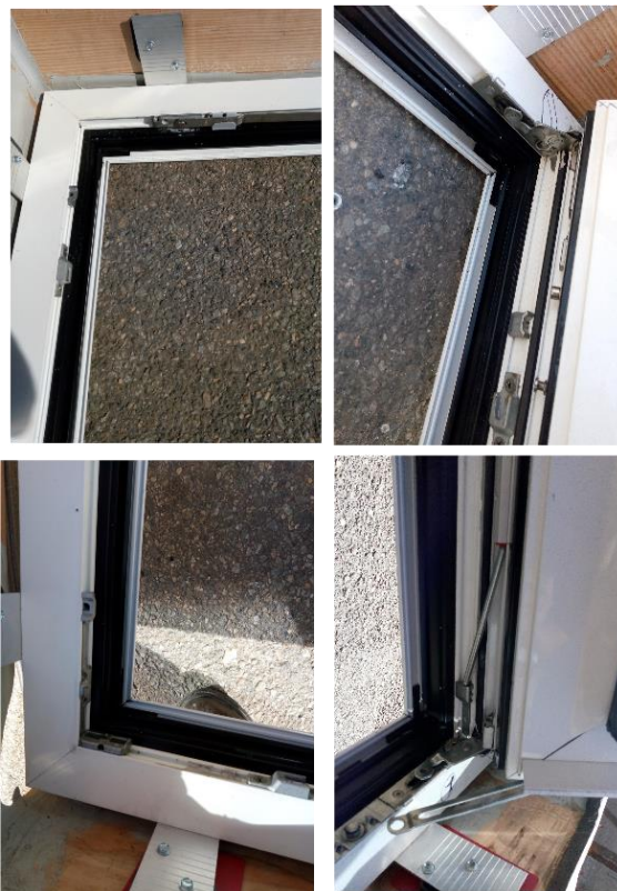
Photo No. 5 Views of frame corners with hardware
